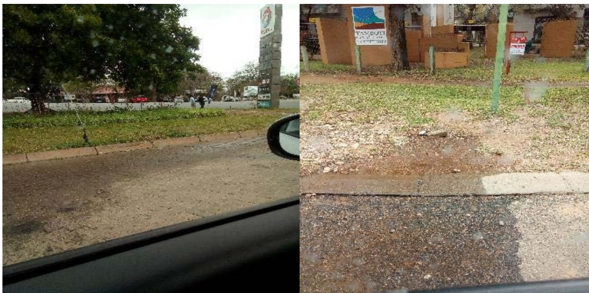
Figure 5: Lack of water management
