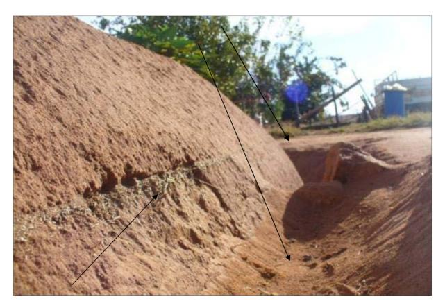
Figure 3.5: Water mark against the ridge above the long <u>bottom ditch</u>. Water overflowed safely out of the ditch (downhill, to the right on the photo) once the water reached this level.
