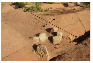
Figure 3.4: Escape routes for excess rainwater flows: (1) escape spillway and (2) the long bottom ditch.
