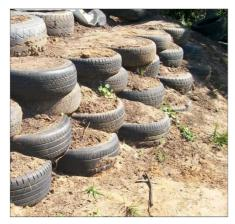
Figure 4.11: A terrace built easily and cost-effectively using old tyres packed with soil.
