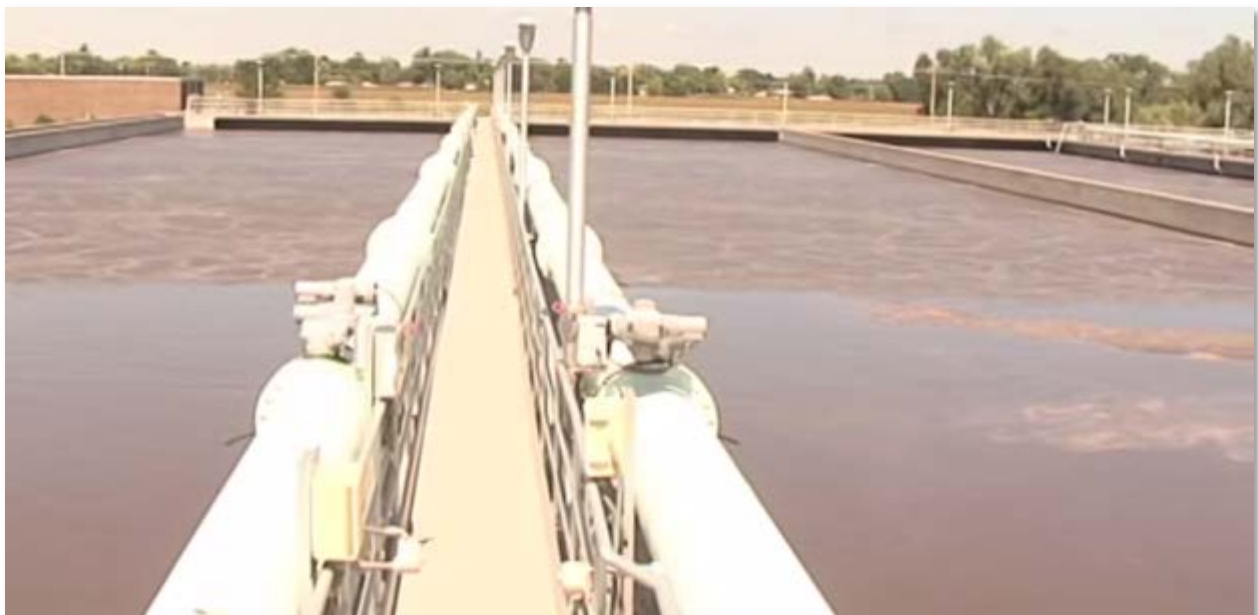
Figure 9: Anoxic and oxic zones of an aeration chamber (SOURCE: https://www.youtube.com/watch?v=pRaptzcp9G4 )
