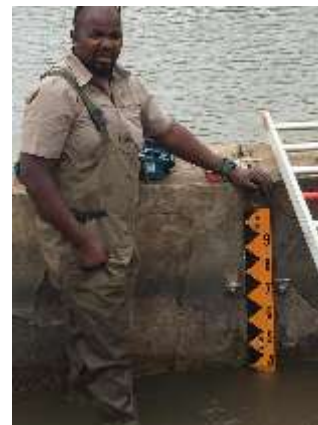
Figure 10: Replacing the gauge plate at Oxford weir.
