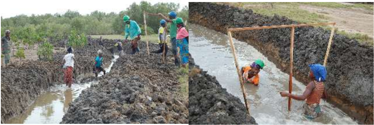
Figure 6: Community participation in channel excavation to restore water flow to the mangroves.
