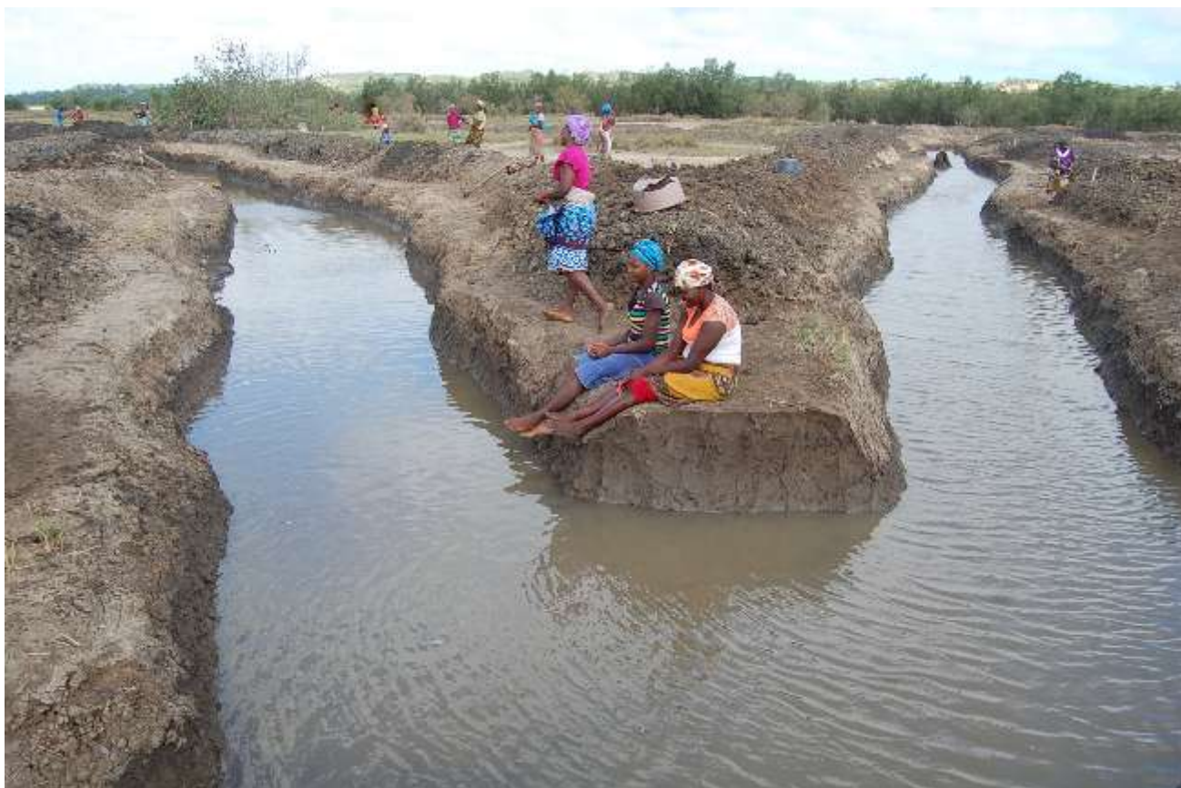
Community participation in restoring hydrological flows to the mangroves in the Limpopo Estuary, Mozambique (Photo credit: CDS-ZC)
